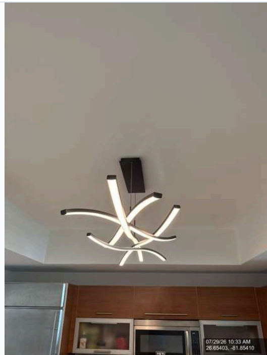
Photo 24 - Kitchen & Laundry - Kitchen ceiling and walls for water stains or moisture
