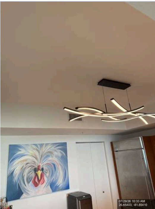
Photo 23 - Kitchen & Laundry - Kitchen ceiling and walls for water stains or moisture
