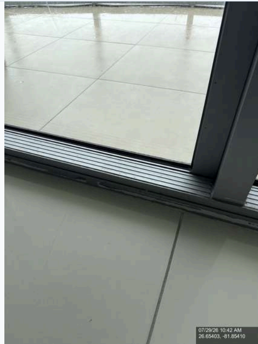
Photo 40 - Interior, Living & Security - Doors, windows, and sliders: damage and proper operation
