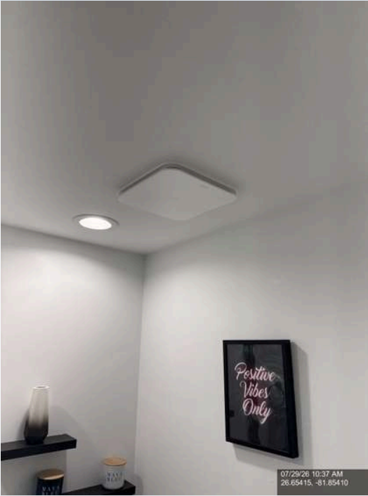
Photo 29 - Baths & Plumbing - Guest bathroom ceiling and walls for water stains or moisture
