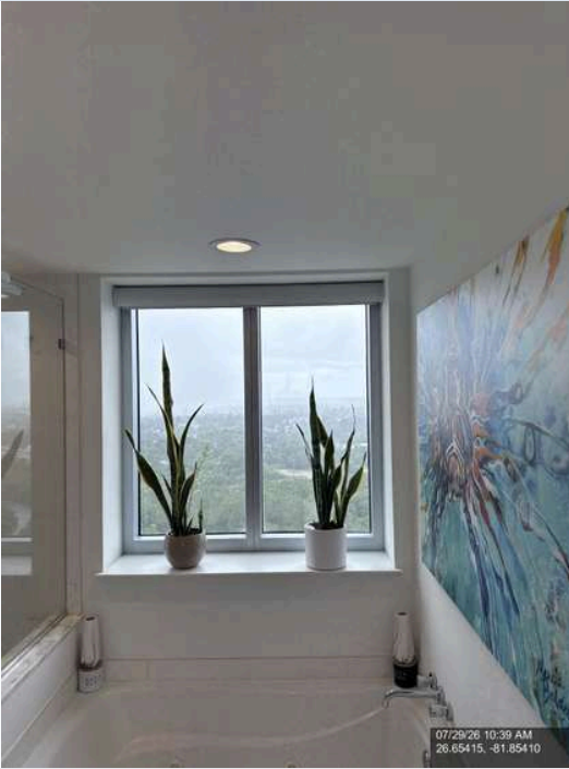
Photo 33 - Baths & Plumbing - Master bathroom ceiling and walls for water stains or moisture
