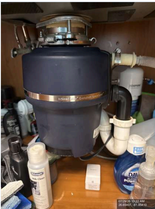
Photo 15 - Kitchen & Laundry - Operate kitchen faucet and check under sink for leaks
