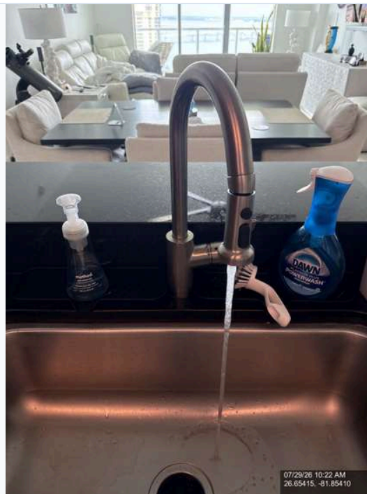
Photo 14 - Kitchen & Laundry - Operate kitchen faucet and check under sink for leaks
