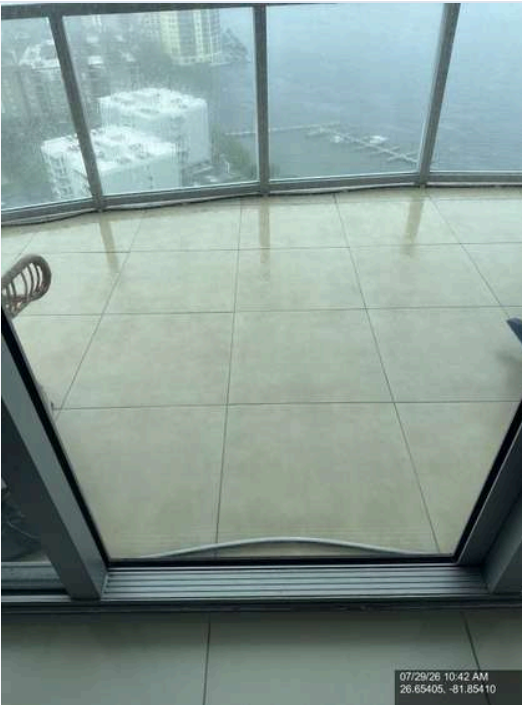
Photo 39 - Interior, Living & Security - Doors, windows, and sliders: damage and proper operation
