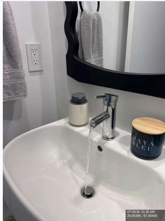
Photo 26 - Baths & Plumbing - Operate all faucets and showers, check flow and drainage
