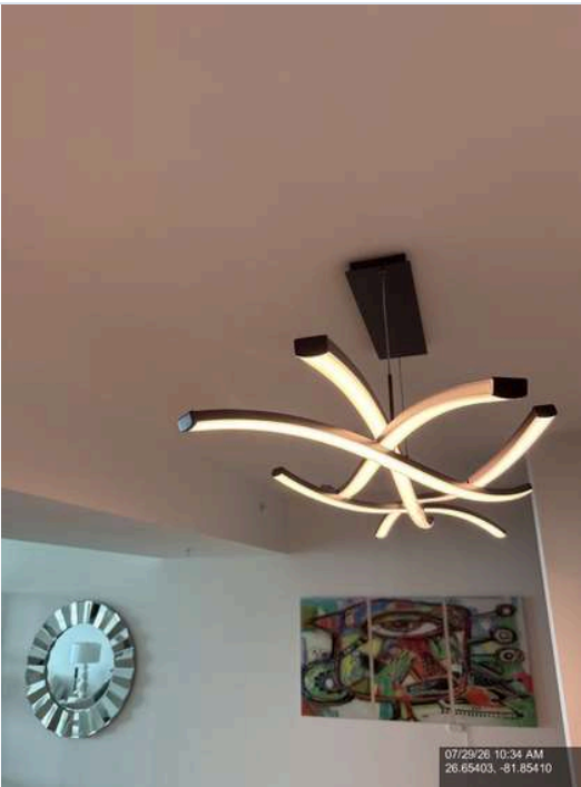
Photo 25 - Kitchen & Laundry - Kitchen ceiling and walls for water stains or moisture
