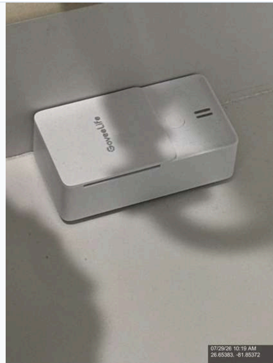
Photo 12 - Mechanical & Systems - Smoke and carbon monoxide detectors
