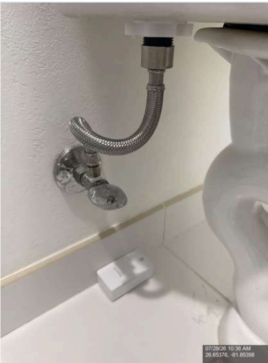
Photo 27 - Baths & Plumbing - Under all sinks and around toilet bases
