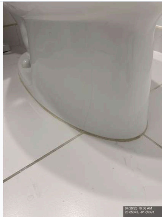
Photo 28 - Baths & Plumbing - Under all sinks and around toilet bases
