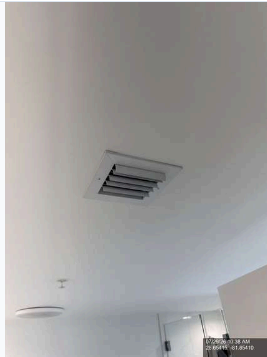
Photo 32 - Baths & Plumbing - Master bathroom ceiling and walls for water stains or moisture
