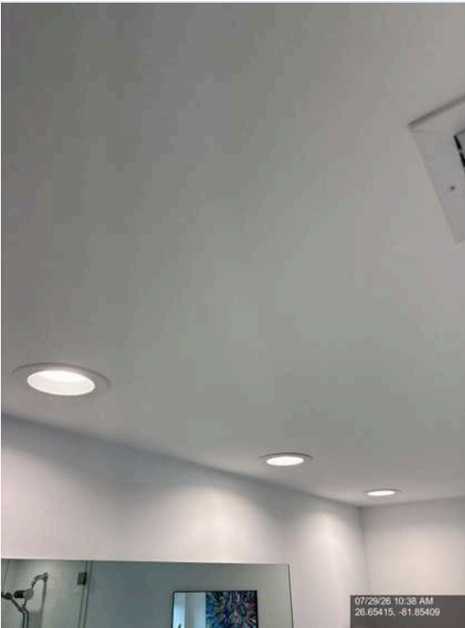
Photo 31 - Baths & Plumbing - Master bathroom ceiling and walls for water stains or moisture
